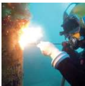
Gambar 1 Under Water Welding
